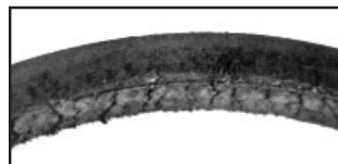
Weathering or "Crazing" Cause: Belt drive elements, as well as aggravation by small sheaves. Remedy: Check tension, provide drive protection and replace belt(s).
